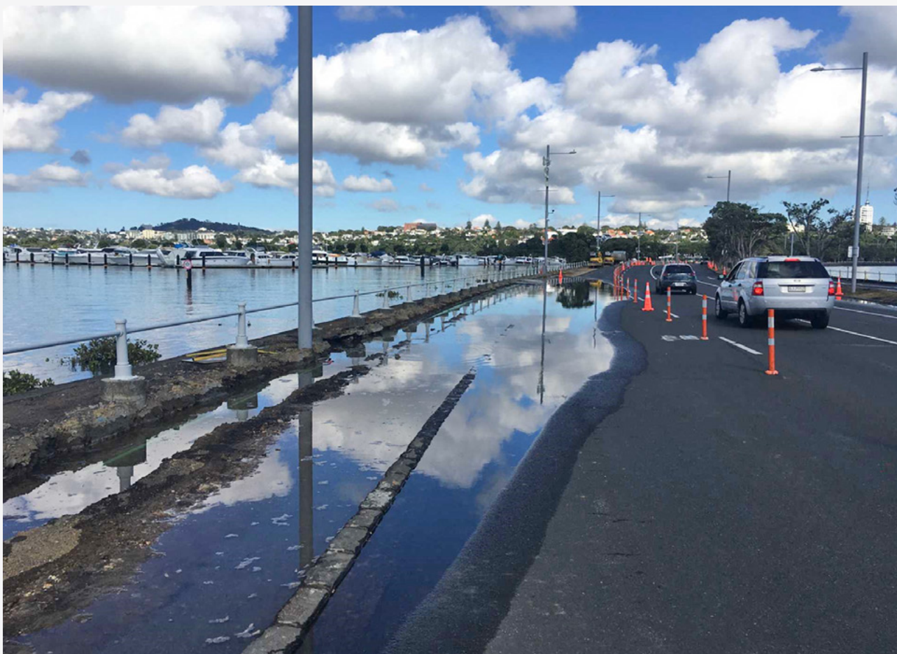
► Blue sky flooding from a king tide on Tamaki Drive, Auckland, March 2020.
